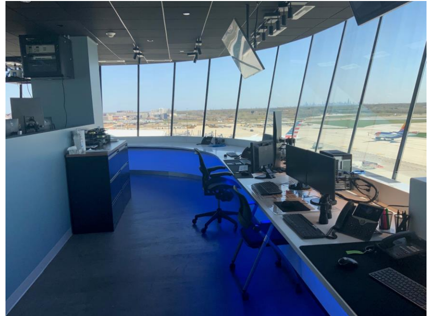
East Extension Ramp Control Tower
